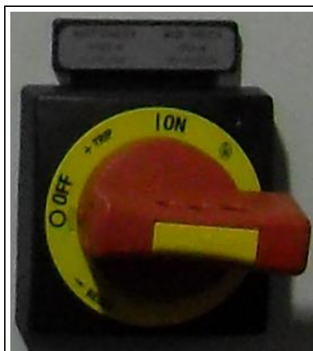
Figure 7: Mains isolation
